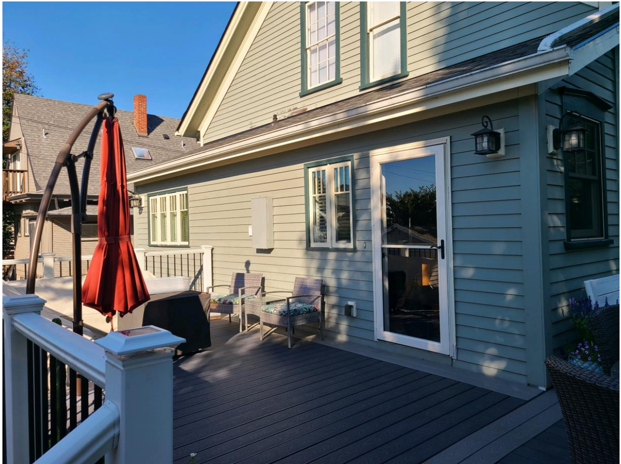
Figure 3- Existing rear elevation showing new deck and 1990s rear enclosed porch addition.
