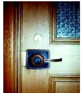
This door handle has been retrofitted to meet ADA requirements. Photo: NPS files.
