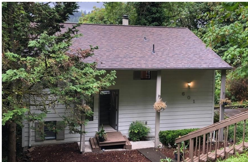
Figure 2. Before new siding and porch rail
