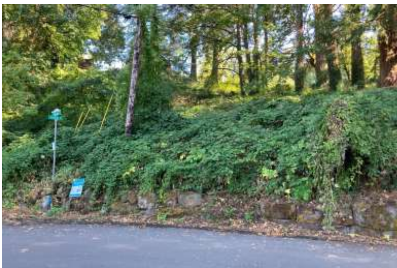
4 th Avenue rock wall existing conditions.
