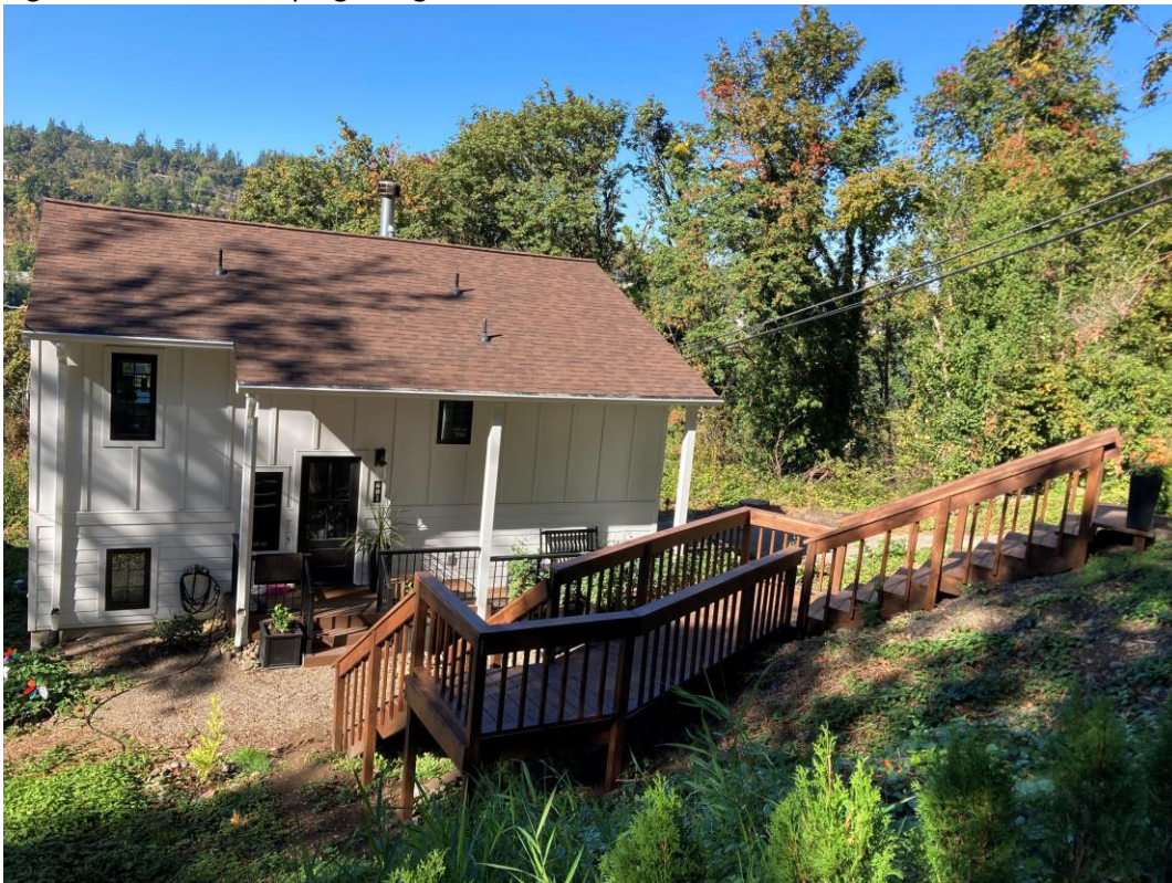
Figure 6. New staircase in front yard
