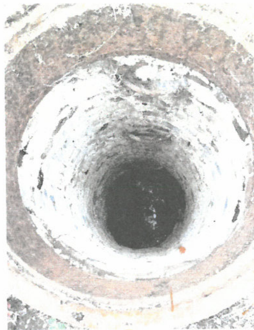
Figure 4-1. Historic brick manhole along the Singer Creek alignment
