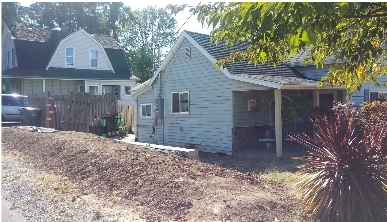
House Currently. Side view from John Adams St. You can see what is left of the 6ft fence that needs to be replaced.
