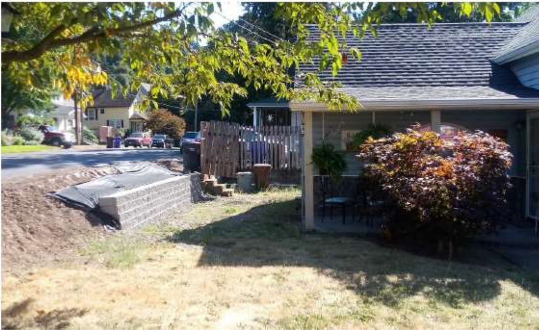
House Currently. Front view from 4th st.
