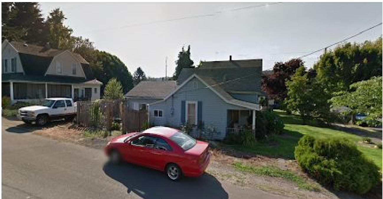
House in 2012 showing the 6ft fence. We would like to extend the fence to our front porch.
