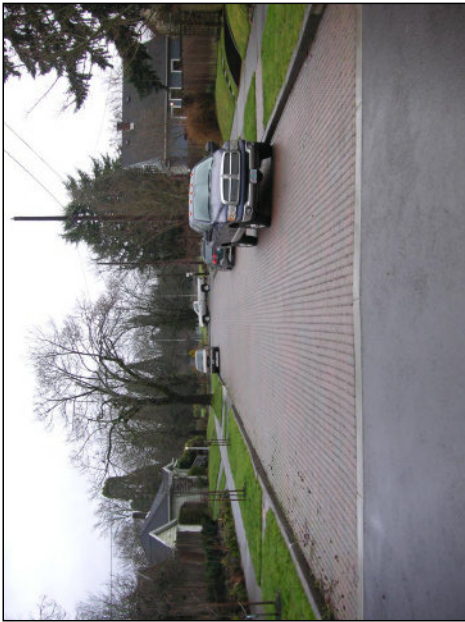
permeable pavers for parking strips and full road treatments
