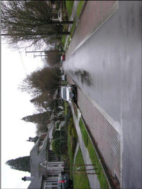
permeable pavers for parking strips and full road treatments
