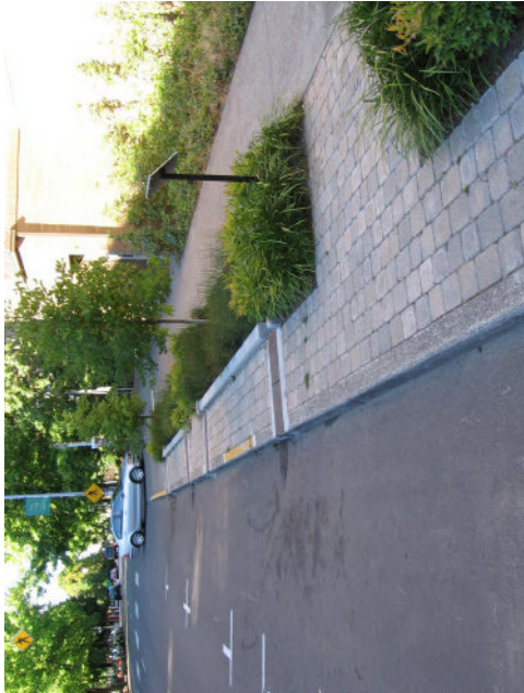
permeable pavers for parking strips and full road treatments
