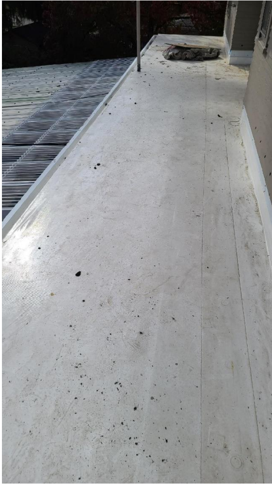
Figure 6. Roof work on rear porch.
