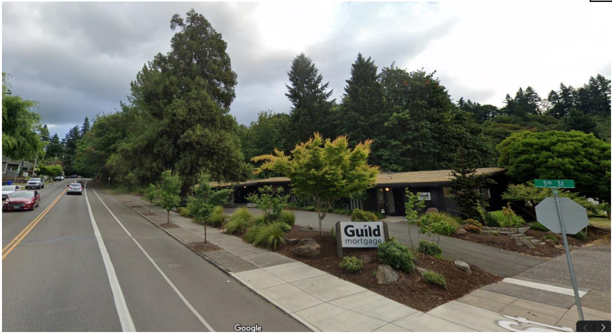
Figure 5 Neighboring building at 1010 5 th Street; a modern commercial building with a low shed roof, roughly U-shaped. The offices are sited in the eastern portion of the building, with a small courtyard framed by the low roof on the west side. The building is primarily clad with stone veneer, but some portions have vertical groove plywood siding. The windows are fixed aluminum sash and are located primarily on the east and west sides of the building. It is not a designated structure in the Mcloughlin Conservation District. (Google Maps- taken prior to construction)
