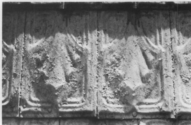
Tin shingles, commonly embossed to imitate wood or tile, or with a decorative design, were popular as an inexpensive, textured roofing material. These shingles 8\frac{3}{8} inch by 12\frac{1}{2} inch on the exposed surface) were designed with interlocking edges, but they have been repaired by surface nailing, which may cause future leakage. (Ballard House, Yorktown, Virginia, photo by Gordie Whittington, National Park Service)
