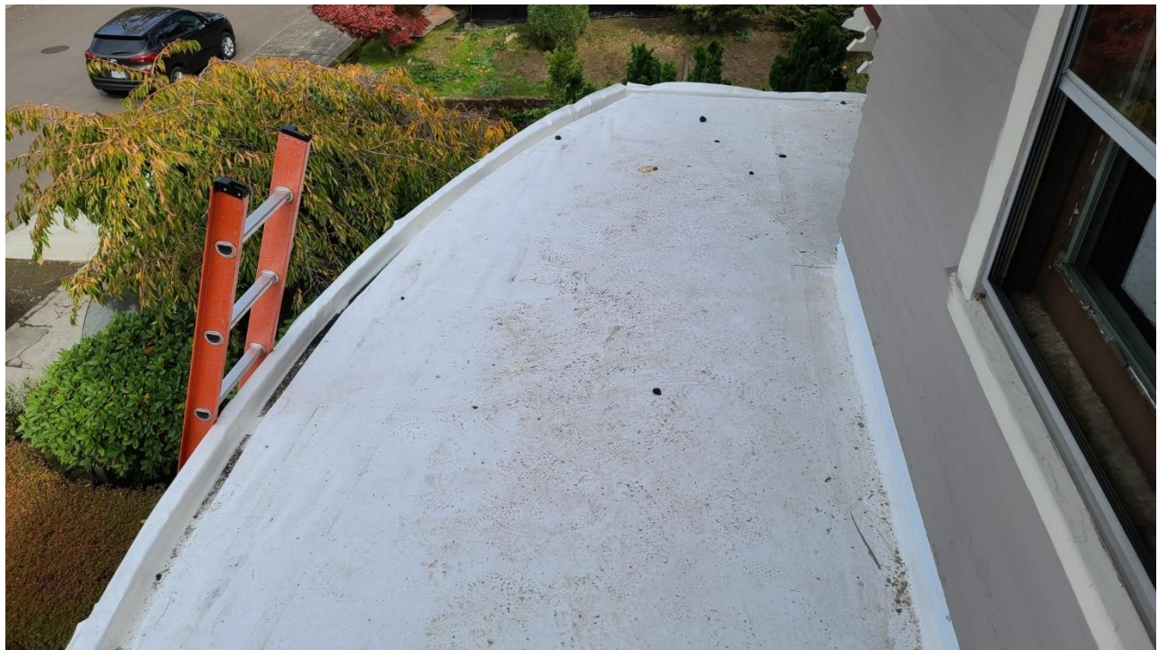
Figure 5. Roof work partially finished on front porch
