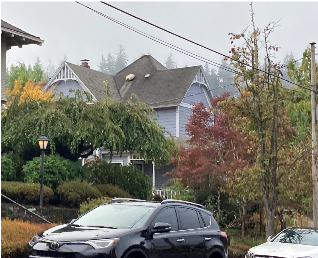
Figure 3. View of roof from Jefferson Street sidewalk (across from 610 Jefferson)
