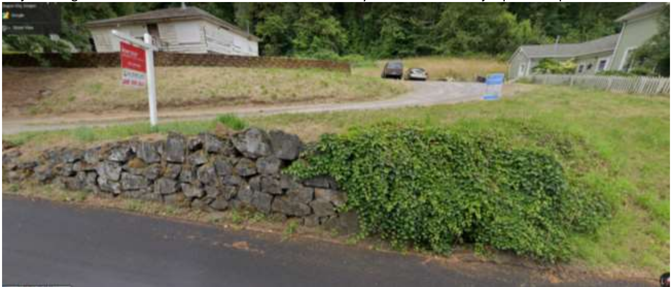
Basalt stone retaining wall in 4 th Avenue right-of-way
