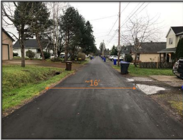
Figure 2-5: Narrow Roadway (Hiram Ave)
