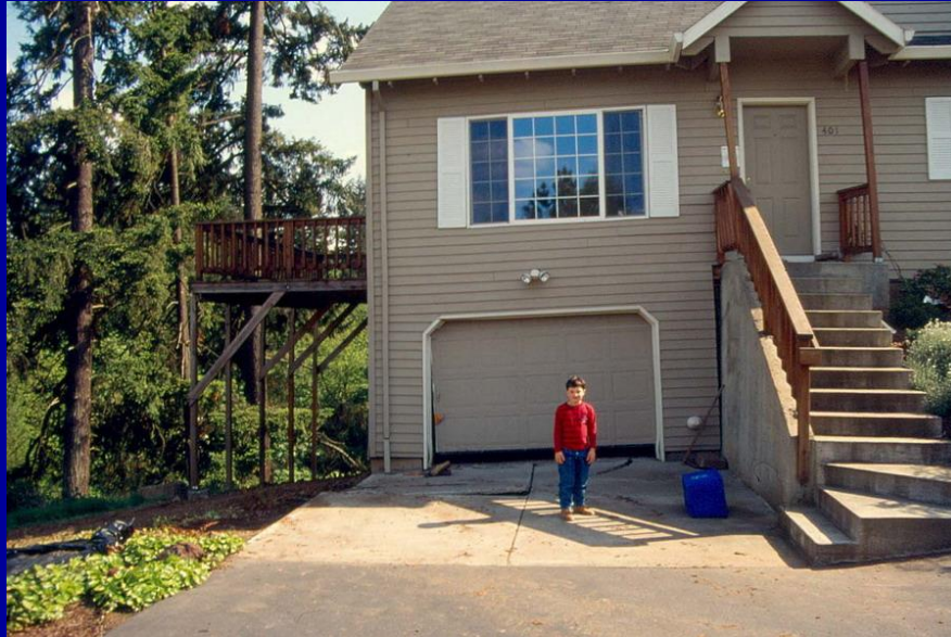
Building on the scarp
