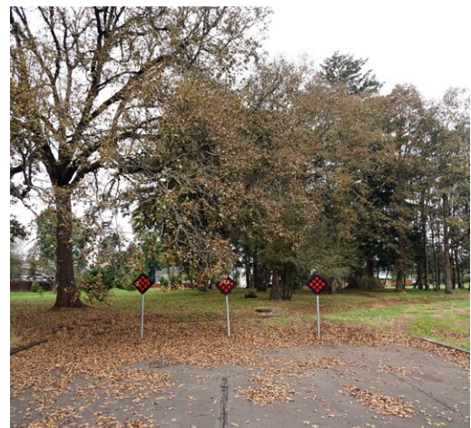
South entrance - ADA access
