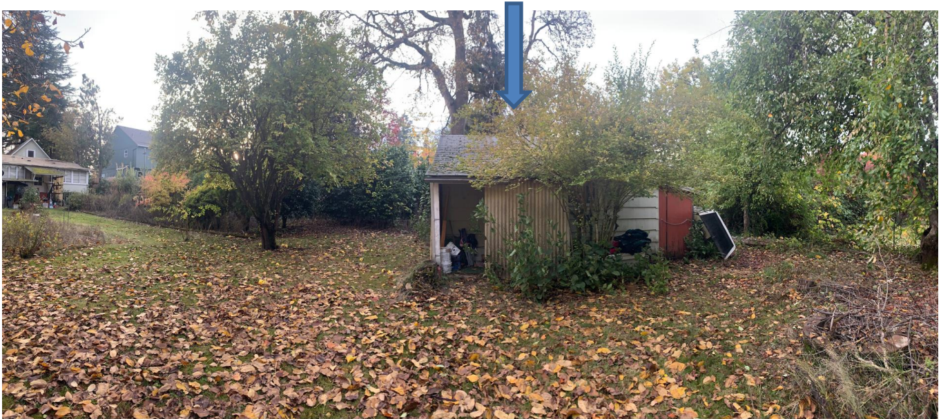
FIGURE 7 LOOKING WEST AT REAR OUTBUILDING
