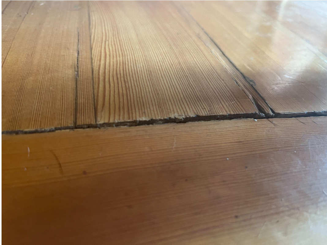
PHOTO A: Lifted Floorboards
