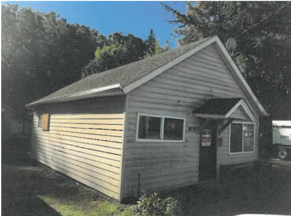
Existing Conditions- front elevation
