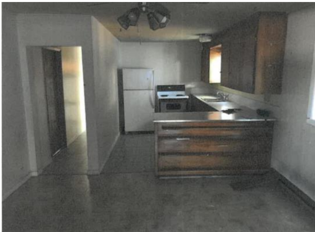
Existing Conditions- interior- kitchen
