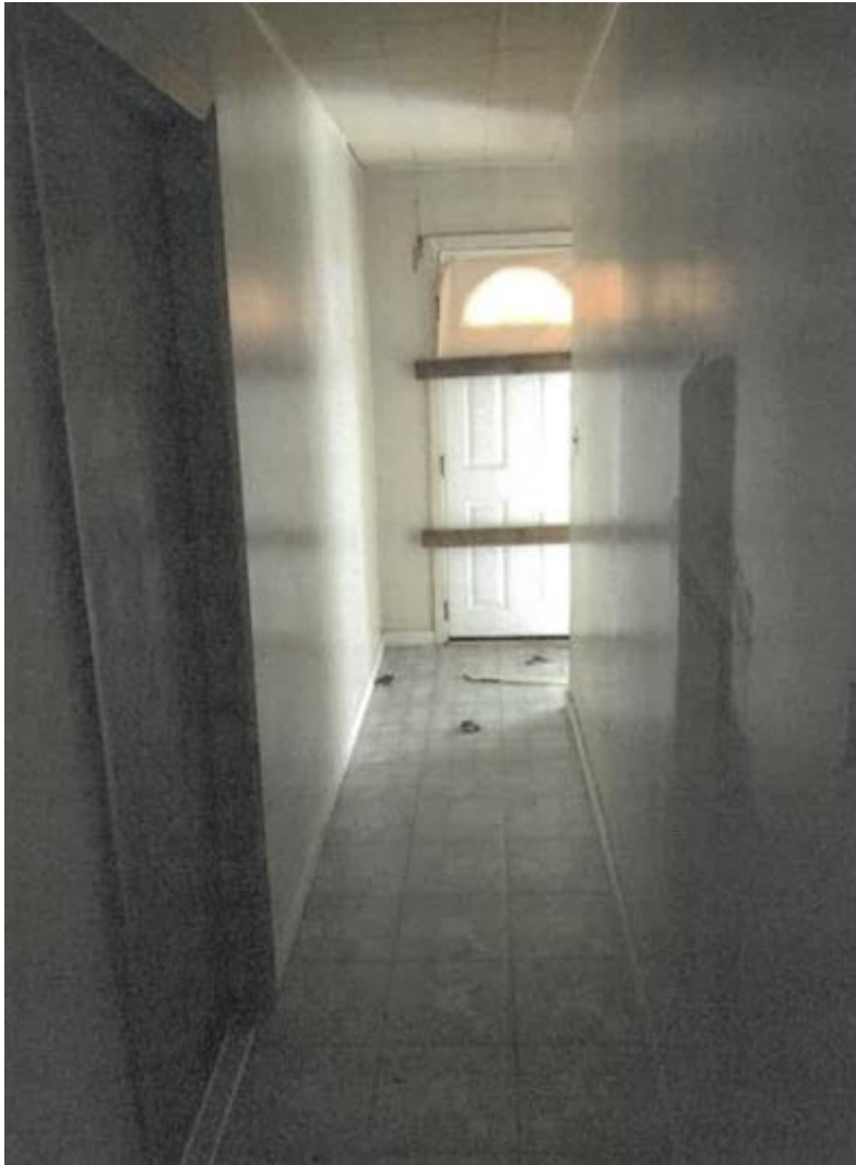
Existing Conditions- hallway to rear porch
