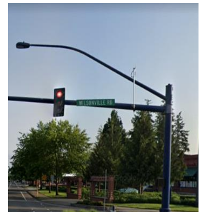
Figure 13: Example of Lighting Upgrade from Acorn to Luminaire at Wilsonville Road/Boones Ferry Road
