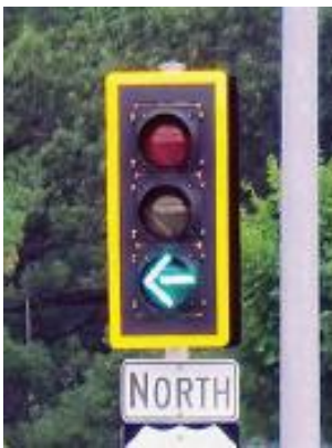
Figure 9. Example Vehicle Signal Backplate with Retroreflective Border
