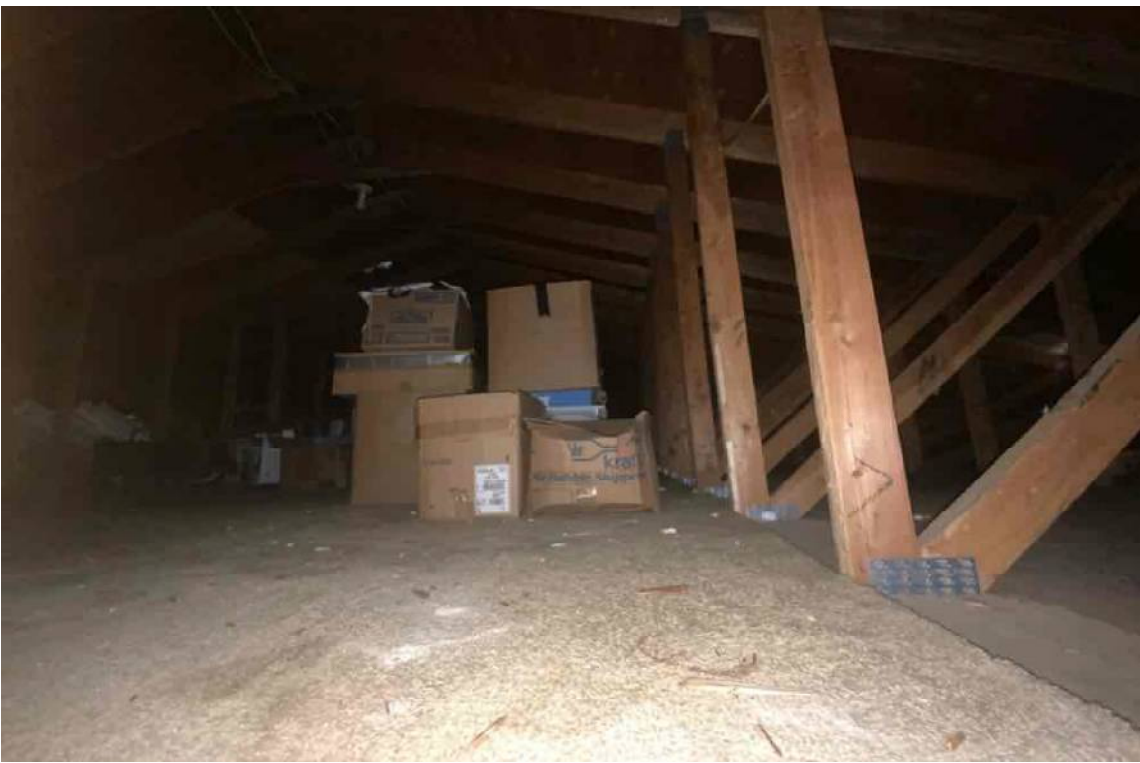
Garage Storage area
