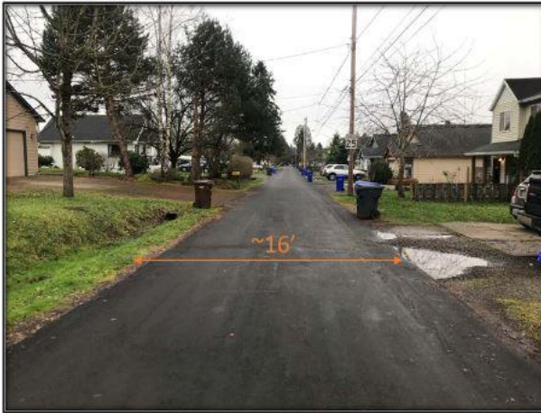
Figure 2-5: Narrow Roadway (Hiram Ave)
