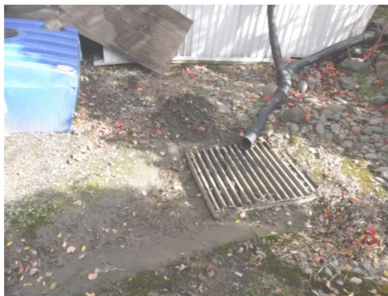
Photo 3-E: SW Catch Basin and Septic Holding Tank (blue).
