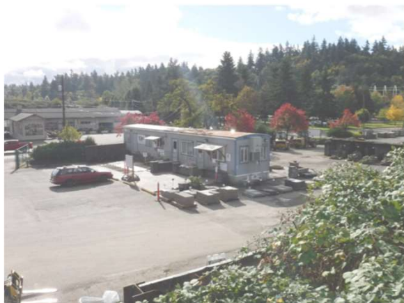
Photo 3-A: Mobile Trailer Type Building on Subject Property.
