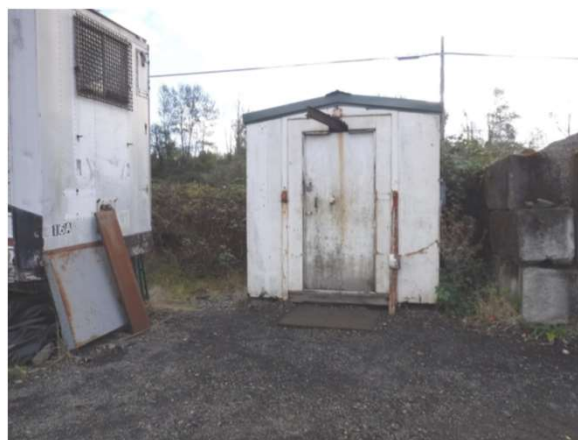
Photo 2-E: Small Maintenance Supply Shed (Petroleum Products Storage).
